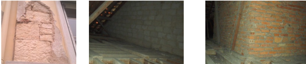
Figure 2.1. Photos of the different walls in the ‘Placa’ Buildings (rubble masonry, concrete blocks and solid and hollow brickwork).
