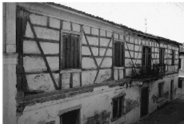
Figure 2-37: Typical morphology of timber-framed masonry infill walls of Lefkas island, Greece [Vintzileou, 2007]
