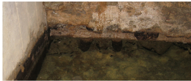
Figure 2-13: Two foundation piles under water
