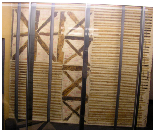
Figure 2-27: Details of the “frontal” walls covered with lath in a building in Guimarães
