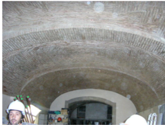
Figure 2-15: Photo of brick groined vault on the ground floor
