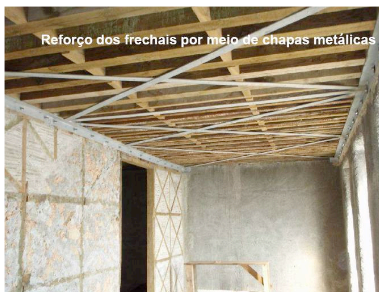
Figure 6-24: In-plane stiffening with metallic diagonals and reinforcement of connection floor-wall [picture from Edifer]
