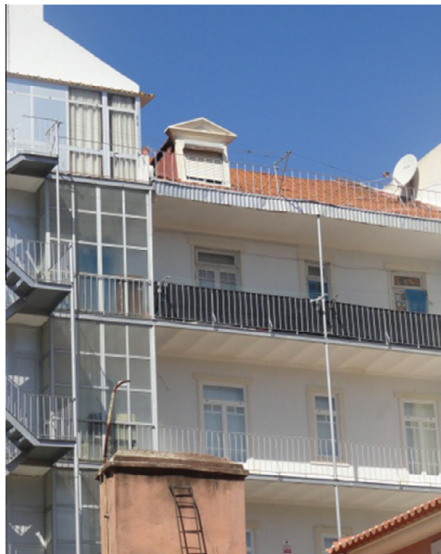
Fig. 3. Steel balcony on the back façade wall.
