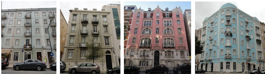
Fig. 1. Typical front façade wall of “Gaioleiro” buildings type I, II, III and IV.
