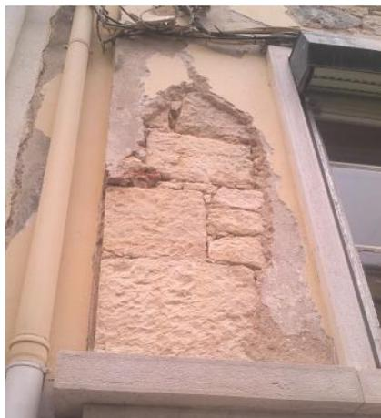
Figure 20 – Photograph taken during the repair works of the façade, on the building in front, where it can observe little mortar on the middle of the rubble masonry.
