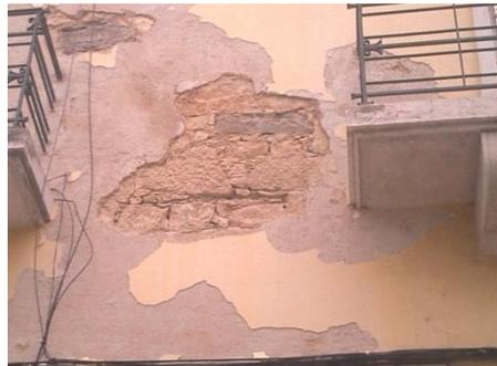
Figure 13 – Rubble masonry walls - Photograph taken during the repair works of the façade of the building in front.
