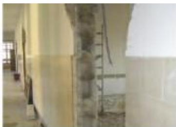
Figure 13 – Voided concrete block interior masonry walls
