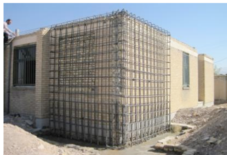
Fig. 31 Photo of the reinforcement of two perpendicular shear walls [Mahdizadeh et al, 2012]
