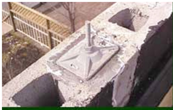
Fig. 27 Close-up view of a post-tensioning anchorage [Ahmad, 2012]
