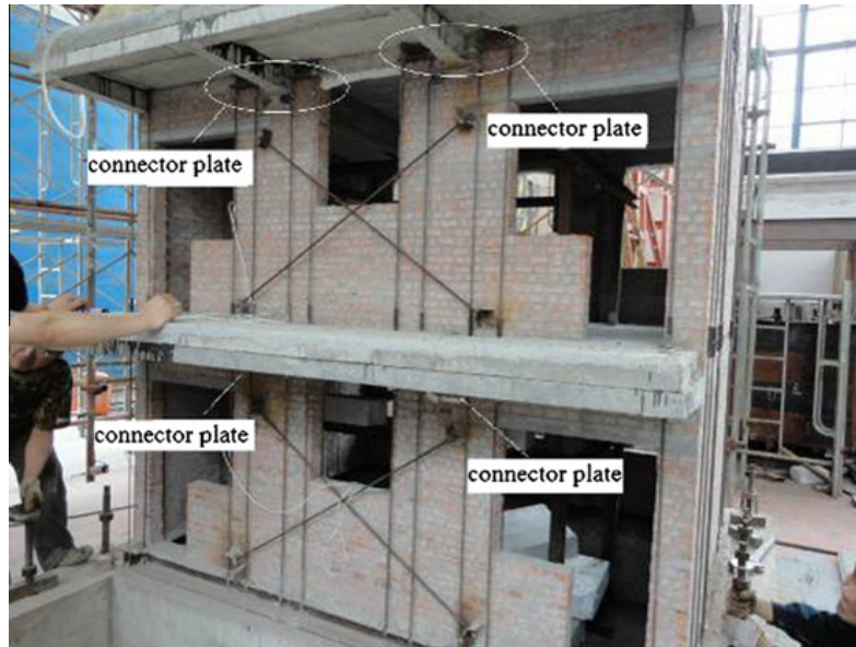
Fig. 28 Cross bracing struts at the first two storeys
