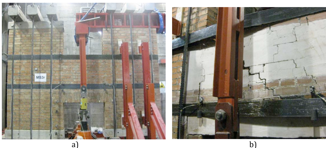
Fig. 18 (a) Wall to be tested in-plane with strengthened spandrels with CFRP (b) view of strengthened spandrel after testing showing debonding of the CFRP [Amadio et al, 2012]
