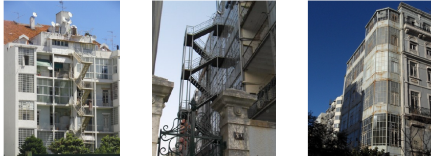
Figure 46 – Steel service stairs and galleries on 'gaioleiro' buildings (Andrade, 2011).
