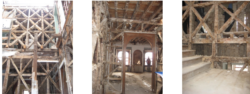
Figure 97 – Structural variations of the 'frontal' walls on the building.
