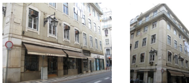
Figure 5 – Limestone blocks on the ground floor façade wall and on the corner of a 'pombalino' building.
