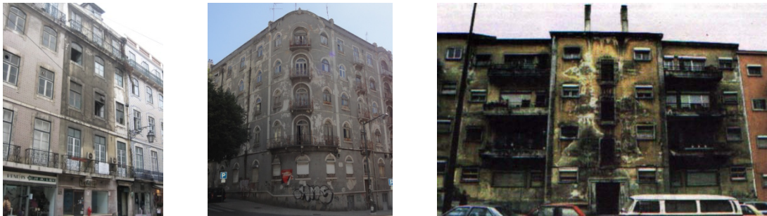
Figure 108 - Degradation of the façade wall of old masonry buildings.
