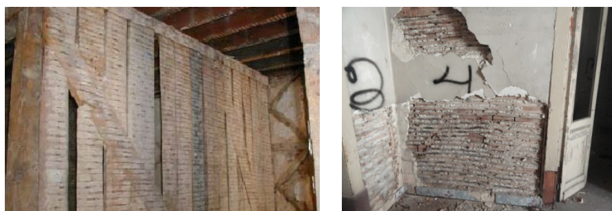
Figure 35 – Example of 'tabique' walls (Pena, 2008).
