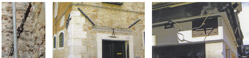
Figure 7 – Iron ties in the connection between orthogonal masonry walls and between parallel masonry walls at the floors level (Lopes et al. , 2008).
