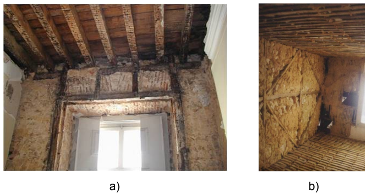
Figure 32 – 'Pombalino' cage (Appleton, 2008): a) Timber frame on the façade walls and relieving arch lintel above the window; and b) Interior timber-masonry walls ('frontal' and timber floors).
