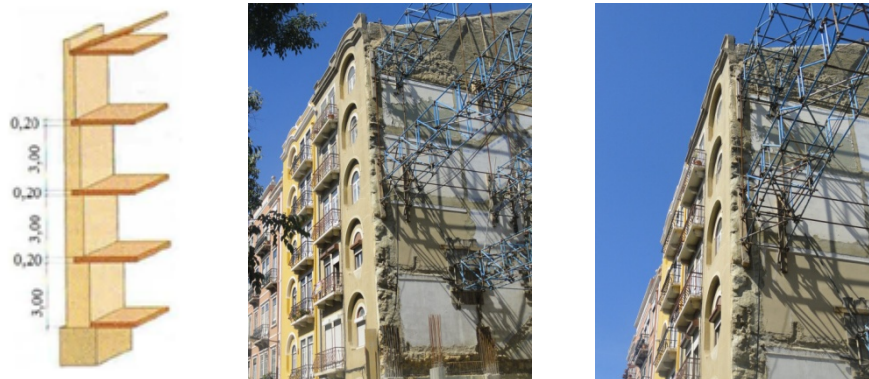
Figure 6 – Reduction of the wall thickness along the height of the building (Appleton, 2003).
