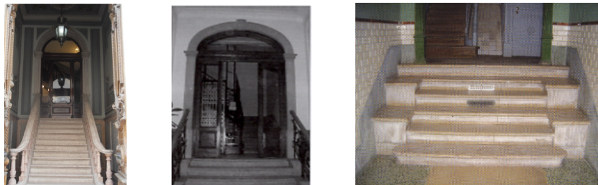
Figure 50 – First flight of masonry staircase gives access to an elevated ground floor with ventilated box underneath (Andrade, 2011 and Appleton, 2005).
