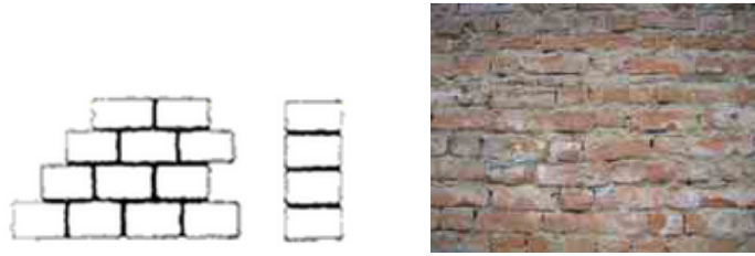
Figure 10 – Brick masonry walls characteristic of a 'gaioleiro' building (Jones, 2002 and Carvalho, 2008).
