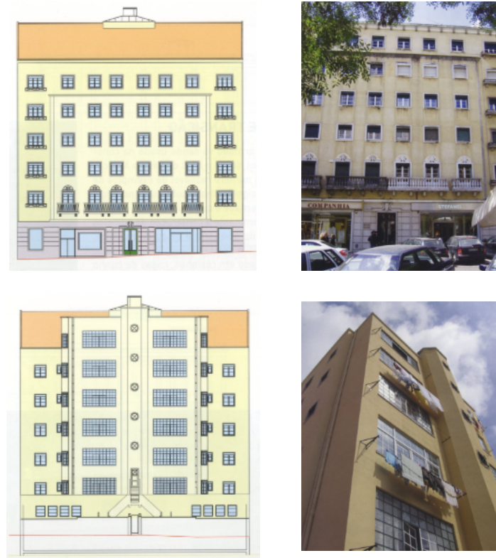
Figure 77 – Front and back façade walls of a 'placa' building in Guerra Junqueiro Avenue (Lopes et al. , 2008). The concrete elements on the façade walls allow larger spans on the ground floor.
