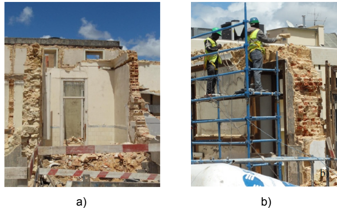
Figure 53 – Brick masonry walls (Andrade, 2011): a) Example of a light-shaft with rubble stone masonry wall (on the left) and solid brick masonry wall (on the right); b) Hollow brick masonry wall.
