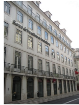
Figure 23 - The windows were aligned both vertically and horizontally in order to maintain the balance of forces (Mascarenhas, 1996).
