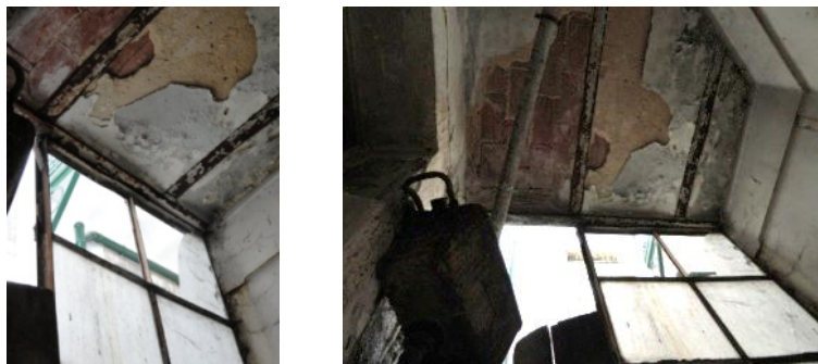
Figure 113 – Oxidation of the steel structure.
