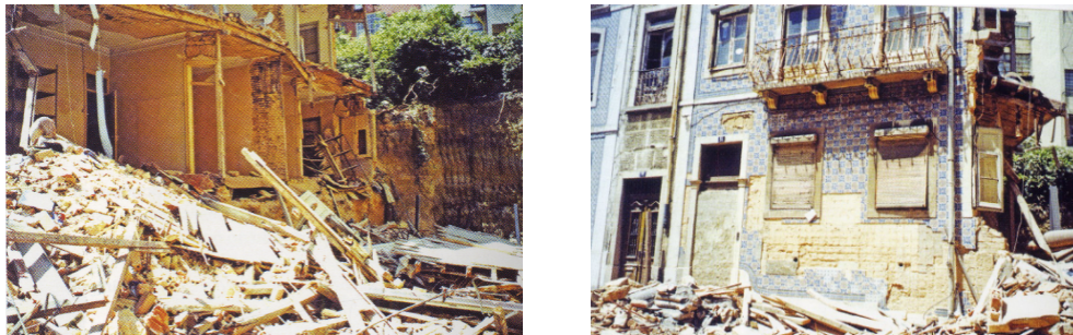
Figure 98 – Collapse of ‘gaioleiro’ buildings (Lopes et al. , 2008).
