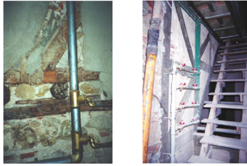
Figure 102 – Cut of a timber joist for the introduction of a pipe, which might compromise the purpose of the ‘pombalino’ cage (Lopes et al. , 2008).
