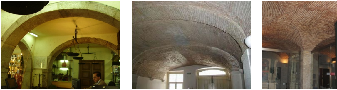
Figure 28 – Example of arches barrel vaults and arches (Appleton, 2003) and crossed vaults.
