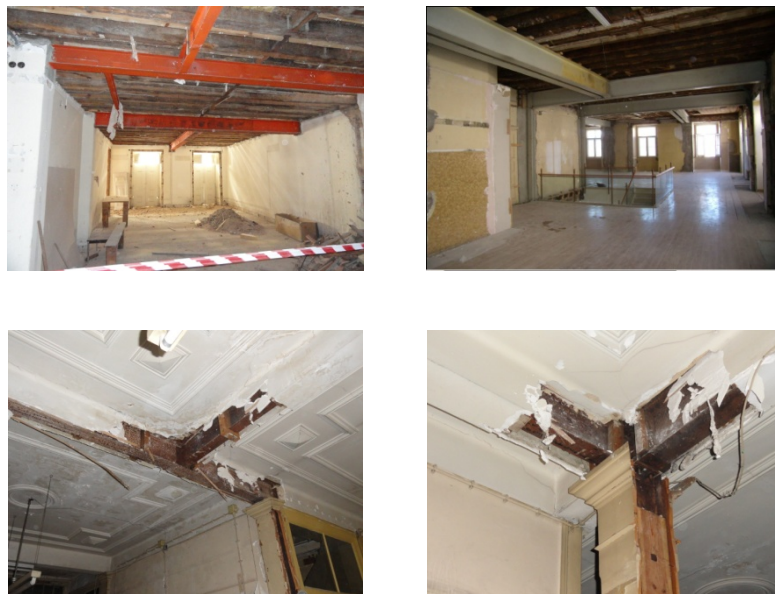
Figure 101 - Removal of interior walls which were replaced by steel beams and columns.
