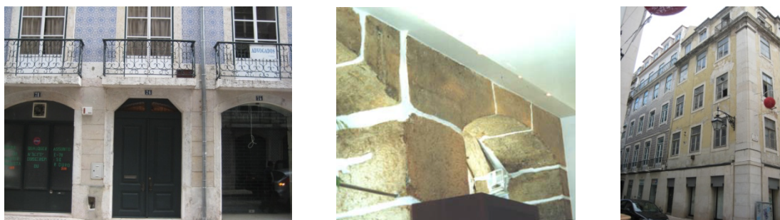
Figure 30 – Ground floor façade wall made of regular limestone blocks.
