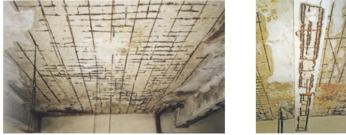
Figure 114 – Reinforced concrete slabs and beams slightly compact concrete with a thin layer covering the reinforcement. The corrosion of the steel is common and leads to the spalling of concrete cover (Lopes et al. , 2008).
