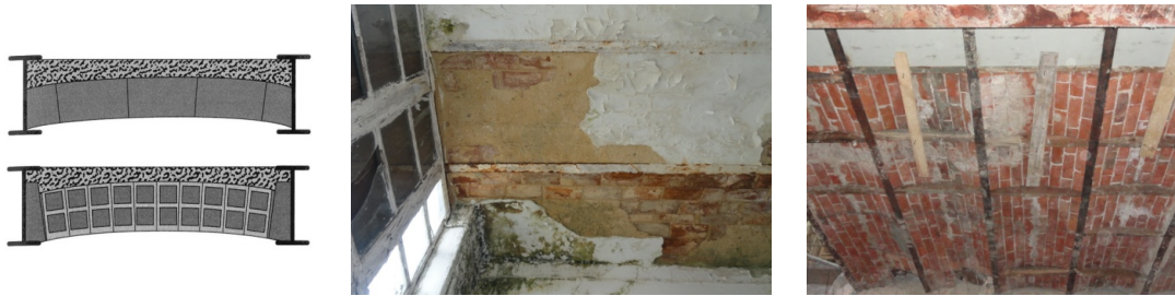
Figure 57 - Floors made of steel beams and ceramic bricks interconnected by mortar or cement (Appleton, 2005).
