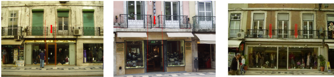
Figure 103 - Example of the interruption of the vertical façade elements.
