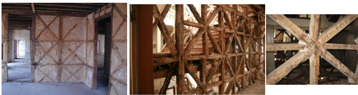
Figure 33 - Example of 'frontal' wall with (Appleton, 2008) and without masonry infill (Lopes, 2010). Despite the regularity that defines the 'pombalino' buildings, there is a great variability in shape and connection of the timber joists.
