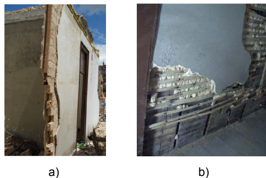
Figure 54 – Interior structure characteristic of ‘gaioleiro’ buildings: a) Solid ceramic brick wall (Andrade, 2011); and b) ‘Tabique’ walls (Pena, 2008).
