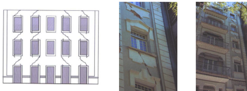
Figure 110 – Diagonal cracking due to differential settlements (Branco et al. , 2011).
