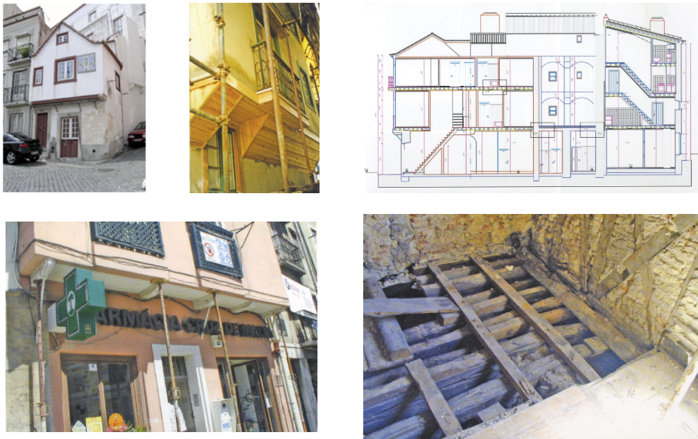
Figure 20 – Buildings from the XVI century with floor ledge and an interior view of the floor with the density of timber beams (Museu da Cidade, 2010 and Lopes et al. , 2008).
