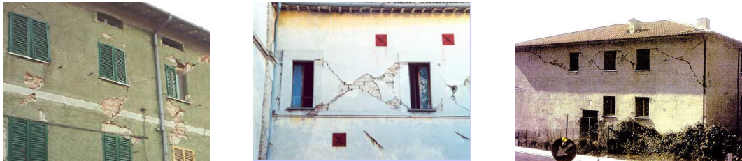
Figure 87 - Damage on a masonry wall around the openings (Logormasino, 2007).
