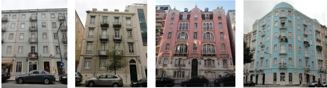
Figure 2. Front façade wall of buildings type I, II, III and IV
