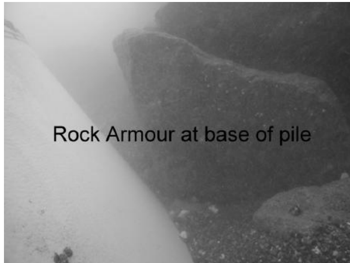
Figure 3.34 – Photographic record of sand and gravel exposure at the monopile wall in Arklow Bank [13].
