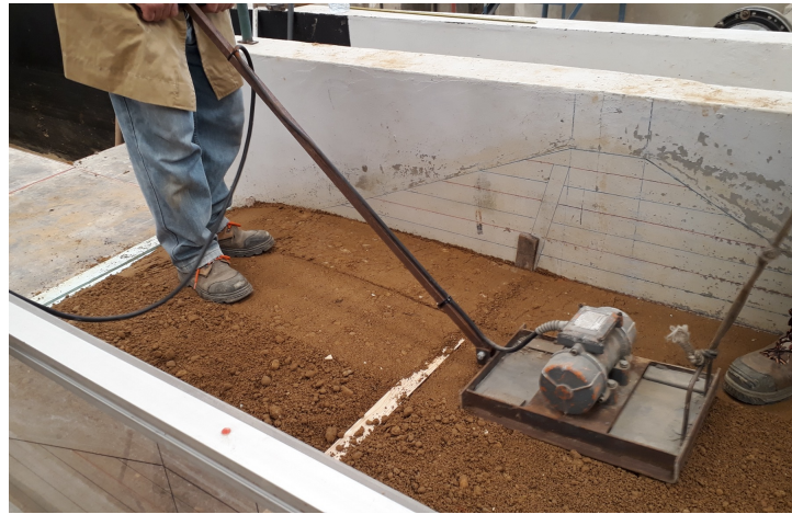
Embankment compaction (5 cm layers)
