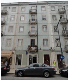
Building 3 (B3) 5-storey Portuguese "Gaioleiro" building (Simões et al. 2013)
