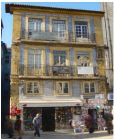
Building 2 (B2) 3-storey limestone Portuguese building (Lovon et al. 2021)
