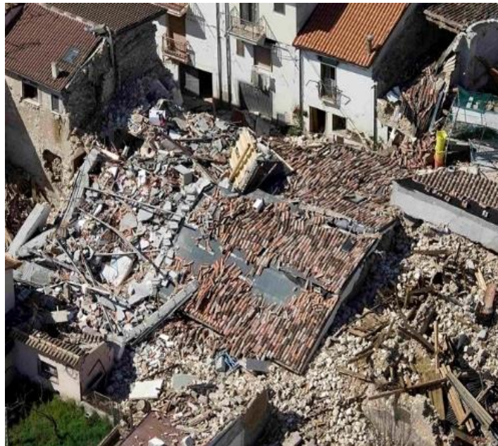
“Zero” collapse mechanism
