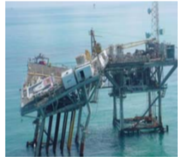
Severe damage caused by hurricane Lilli in the Gulf of Mexico
