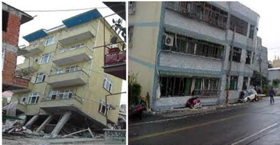
Soft storey failures in Golcuk, Turkey (Izmit and Düzce earthquakes). Source (AIR)
