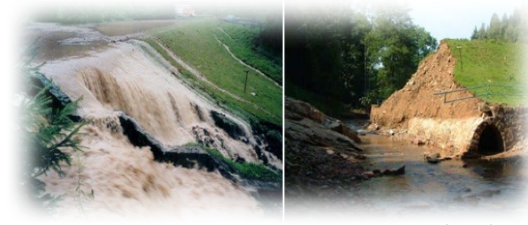
Overtopping and breaching – Glashütte , Germany (2002)
