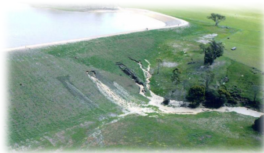
Internal Erosion – Piping – Tunbridge Dam, Tasmania, Australia
