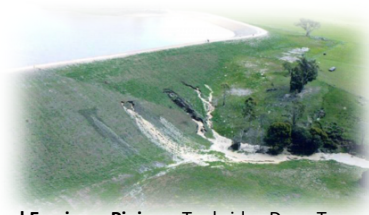
Internal Erosion – Piping – Tunbridge Dam, Tasmania, Australia
