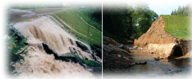
Overtopping and breaching – Glashütte , Germany (2002)
