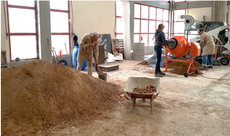
Soil homogenization and humidification
