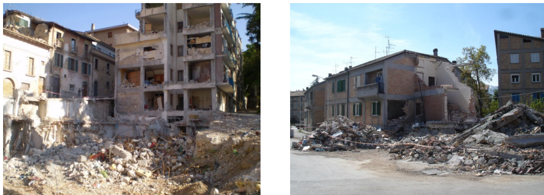
Figure 11.2 – Destroyed buildings after the L'Aquila earthquake [135].
