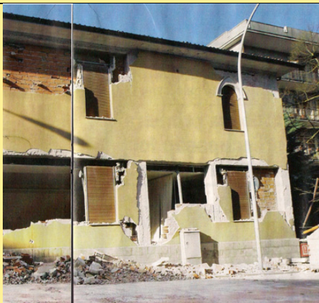
After: Exterior - very heavy damage
