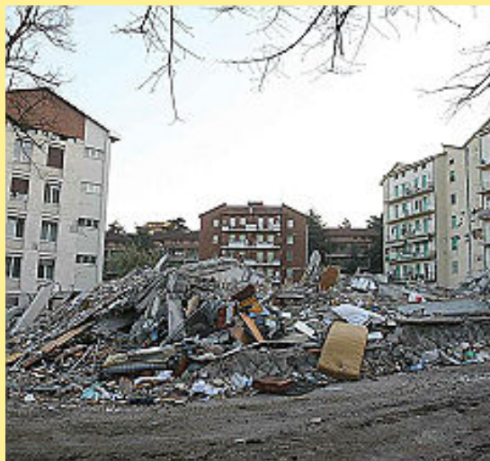
Figure 8: 6-floor reinforced concrete collapse at Via Campo di Fossa , 6 b, L'Aquila.
