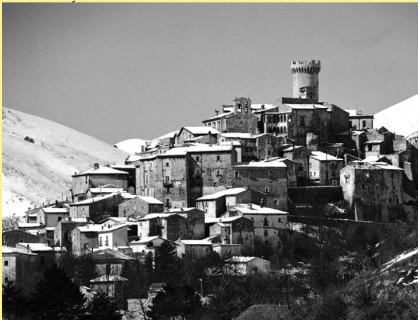
Figure 12: The mountain village of Santo Stefano di Sassanio before the tower collapse.
