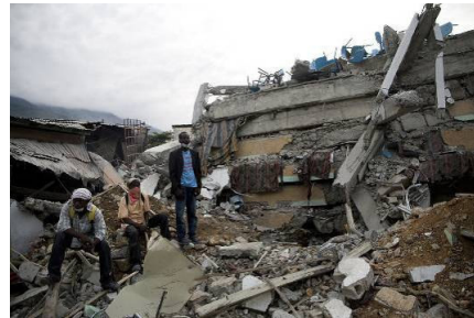
Figure 2. Collapse of the nursing school in Port-au-Prince (left), pancake type collapse of the University of St. Gerard where 200 people died (right)
