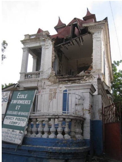
Figure 2. Collapse of the nursing school in Port-au-Prince (left), pancake type collapse of the University of St. Gerard where 200 people died (right)
