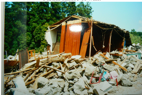
Collapse of masonry walls.
