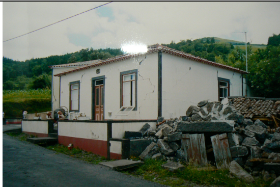
Slight structural damage. Fallen of plaster.
