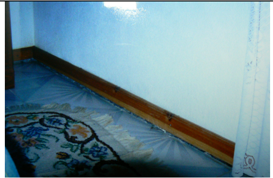
Separation between floor and wall.
