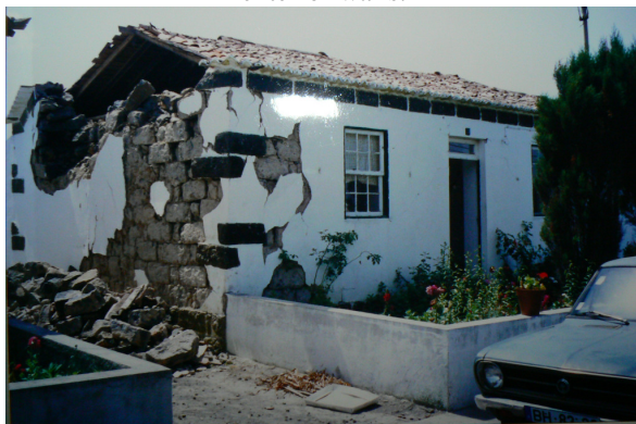
Partial failure of wall.
