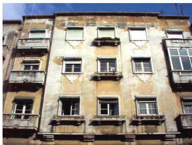
Figure 21 - The masonry buildings with wooden floors prior to 1940
