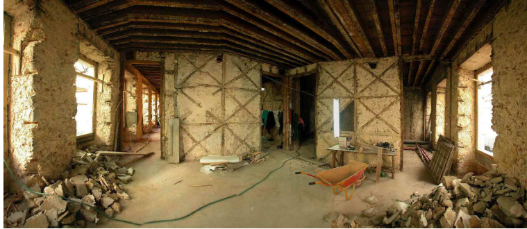
Figure 20 - The "Pombaline" type – "Gaiola". Post 1755 till late XIX th century (photo by R. Langenbach)
