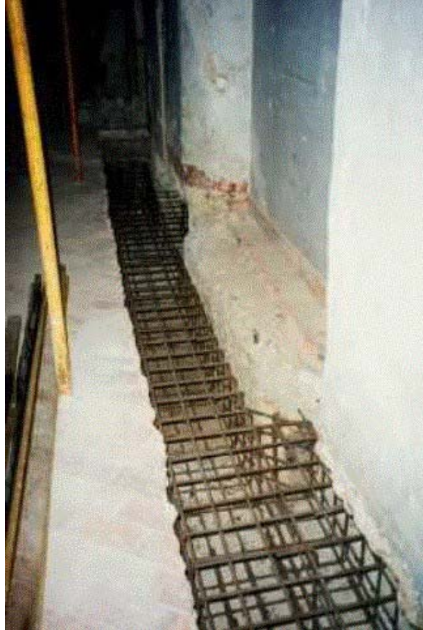
Masonry buildings – structural strengthening with load transfer
