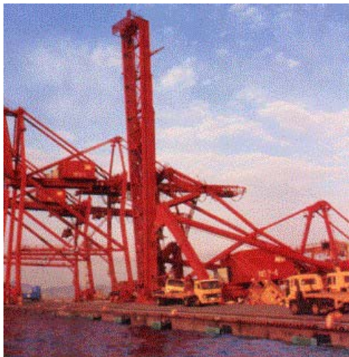
Figure 4 - Damages in equipment at Kobe harbour in Japan, as a result of the earthquake of 17 th January 1995 [3]
