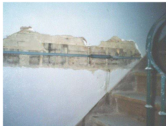
Masonry buildings – applying traditional tie-rods
