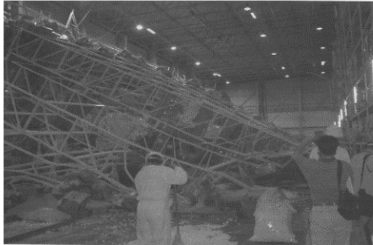
Figure 2 – Fall of the warehouse shelves at the Toprak Ilıc pharmaceutical drug factory
