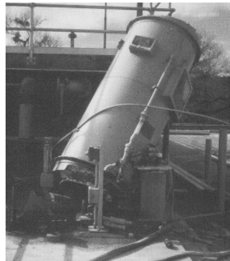
Figure 5 – Fall of air purifying equipment at a treatment plant during the Northridge earthquake, 1994 [4]
