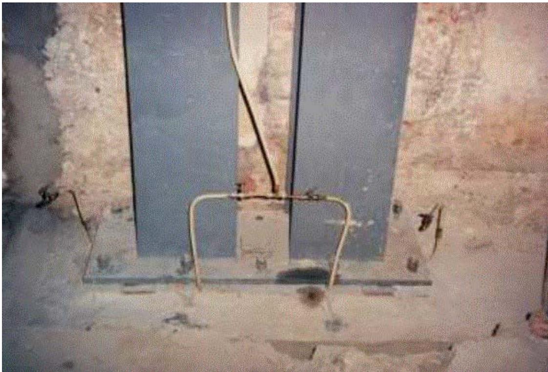
Masonry buildings – structural strengthening with load transfer
