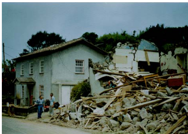
Figure 2 – Difference in the vulnerability in buildings – Faial earthquake, 8 July 1998.
