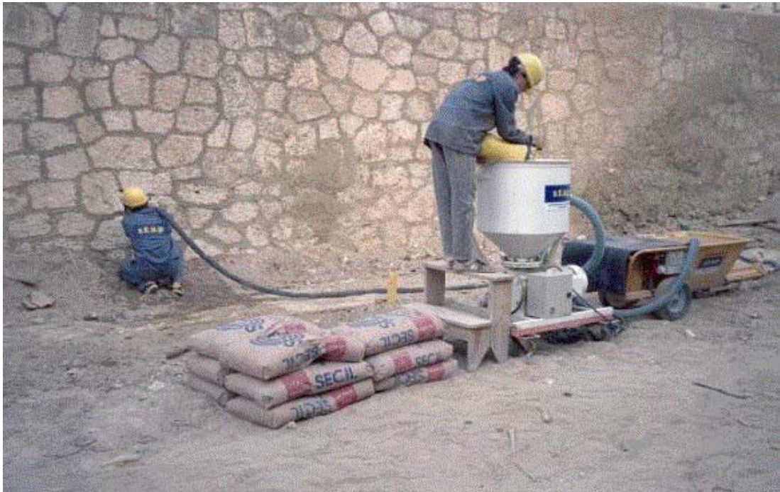
Masonry buildings –grouting
