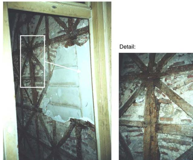
Fig. 3. Timber elements of 'gaiola' enclosed in masonry interior walls.
