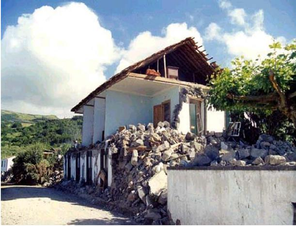
Fig. 4. Fall out-of-plane of the exterior walls without complete collapse (1998 Azores earthquake).
