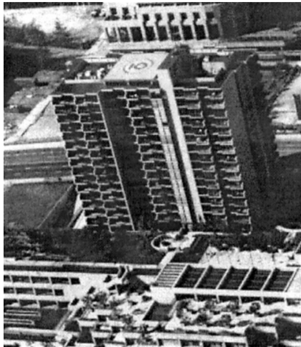
Figure 5. View of Los Angeles 17-storey residential building
