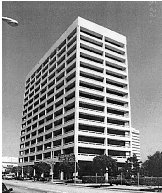
Figure 3. View of Sherman Oaks 13-storey commercial building
