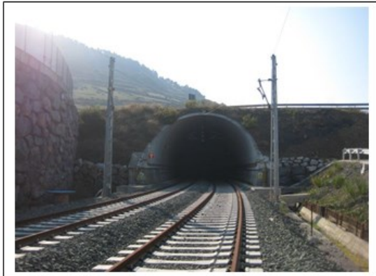
Port side: false tunnel and entrance to the tunnel
