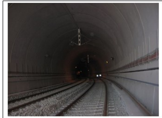
Inside the false tunnel. Please note that the catenaries have not yet been put in place.
