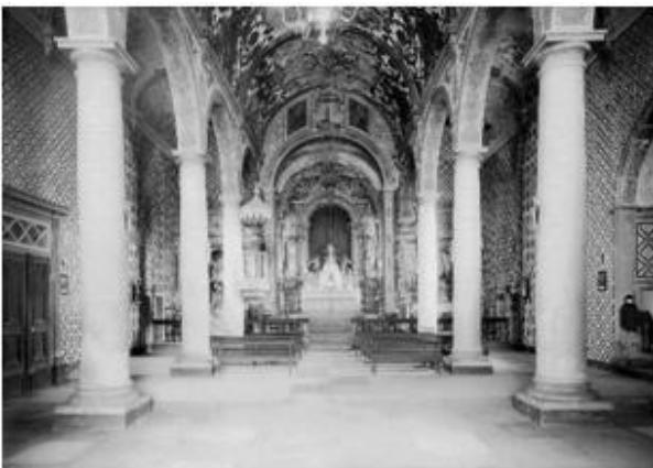
Figure 2 - View of the church interior .Nave and lateral arcades.
