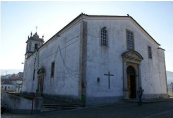
Figure 1 - Bucelas Church. South Wall of the Church. Main entrance)
