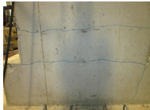
Figure 17. P08.2 rear damage
