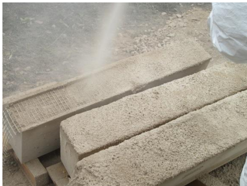
Figure 2. Reinforcement application
