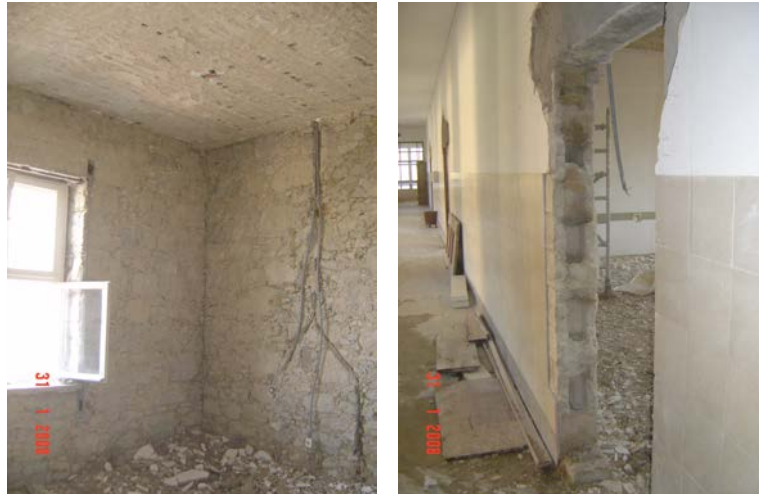
Figure 1.1 Secondary School of D. João de Castro, in Lisbon. Left: rubble stone masonry walls; Right: concrete block masonry walls
