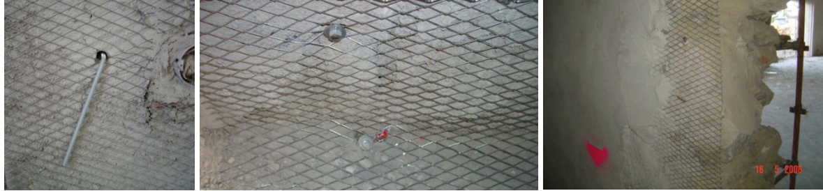
Figure 2.2 Strengthening solution – details of the mesh nailing and anchoring and of the mortar plaster
