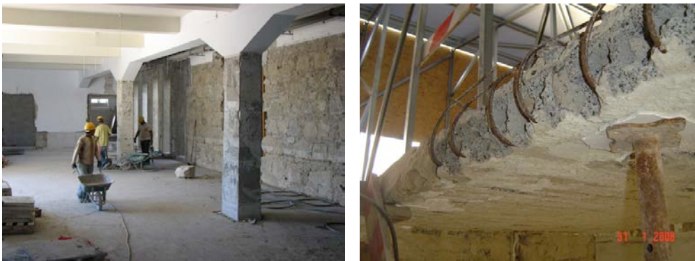
Figure 1.2 Secondary School of D. João de Castro, in Lisbon. Left: reinforced concrete column and beams; Right: Reinforced concrete slab
