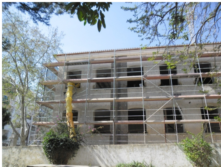
Figure 11. Fibreglass mesh application on the site (exterior leafs) – South elevation
