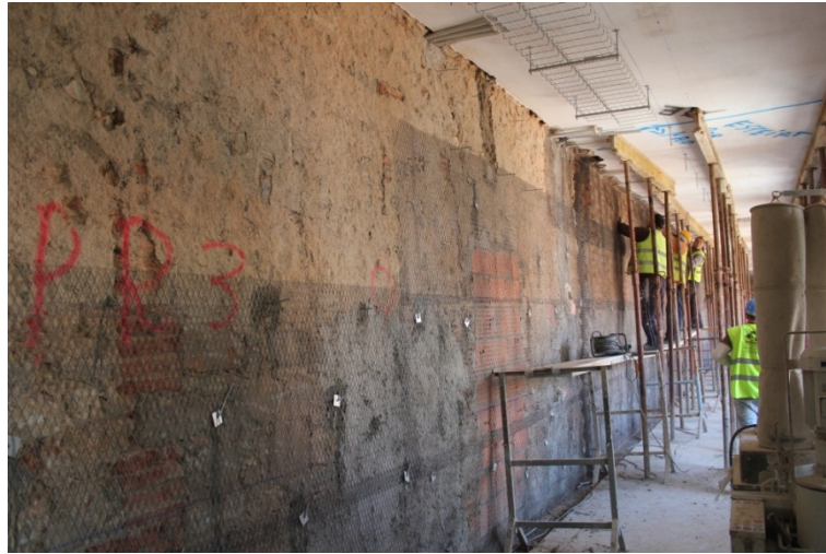
Figure 10. Steel mesh application on the site (interior leafs)
