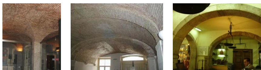
Figure 7. Masonry crossed vaults, barrel vaults (Appleton, 2003) and arches on the ground floor.
