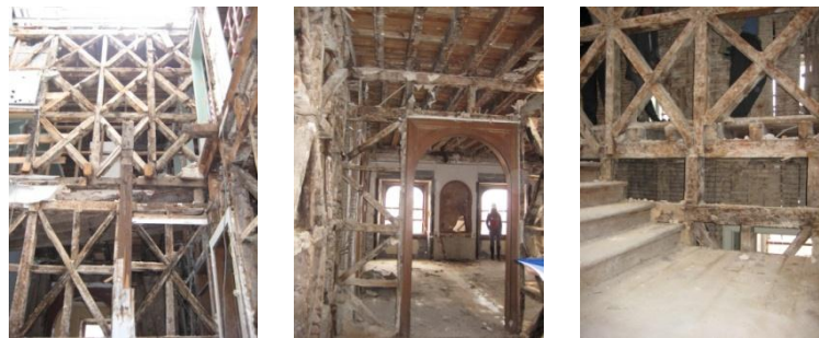
Figure 9. Structural variations of the ‘frontal’ walls on the building.
