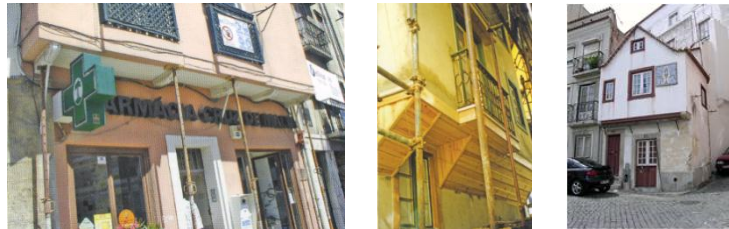
Figure 5. Buildings with rebounded ground floor (Museu da Cidade, 2010) (Lopes, 2008).
