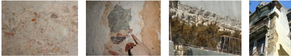
Figure 1. Rubble stone masonry walls.
