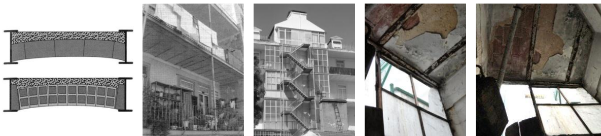
Figure 14. Metallic structures on the back façade wall (Appleton, 2005) and oxidation problems.
