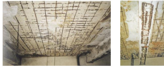
Figure 18. The corrosion of the steel is common and leads to the spalling of concrete cover (Lopes, 2008).
