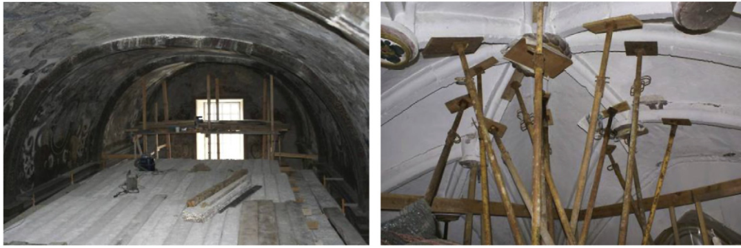
Fig. 1. Damage in vaults due to the removal of the infill. Left: Bucelas Church (Lisbon, Portugal); right: Machico Church (Madeira, Portugal).
