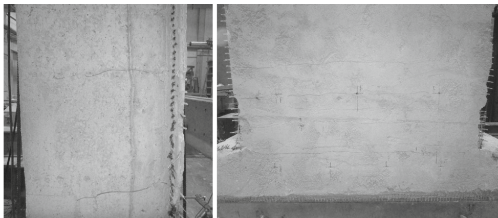
(a) Crack pattern (EPF_01 specimen)
