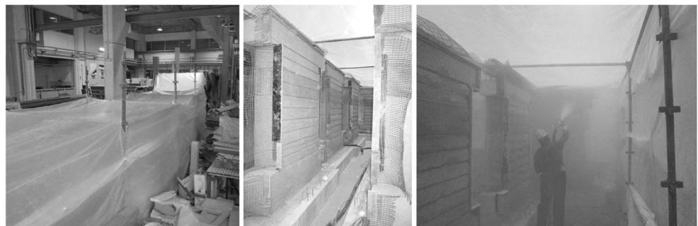
Fig. 2 Render mortar shotcrete operation
