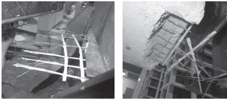
Fig. 9. Damage features of the ECA_01 specimens.
