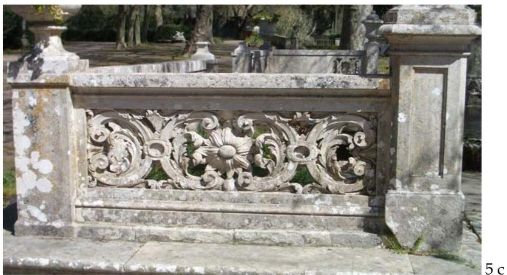
**Figure 5:** Section of the balustrade exemplifying the results of the applied treatments. (a) Before (spring 2006); (b) Fall 2006, five months after application of Preventol 3 % solution; (c) March 2007, six months after application of the zinc acetate solution (1 % Zn).
