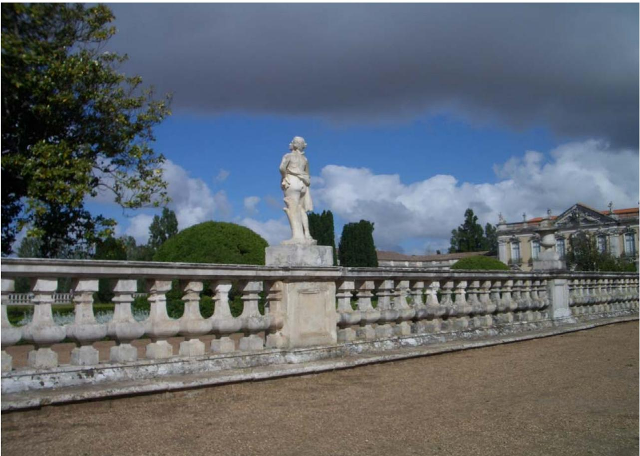
**Figure 7:** View of one of the balustrades in May 2007. The left side was treated in fall 2006. The cleaner appearance of the balusters on the left side is clearly noticeable in comparison to those on the right.
