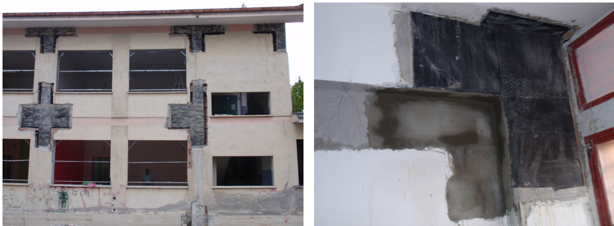
Figure 3. Local strengthening of a reinforced concrete school building in L'Aquila based on carbon fiber
